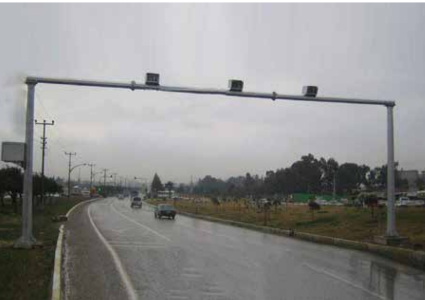
PLATE RECOGNITION SYSTEM CONSTRUCTION
